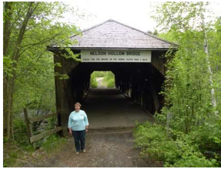
Oldest covered bridge in NB (Nelson Hollow)
